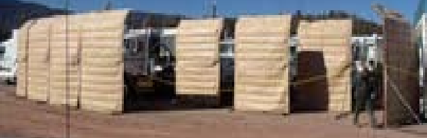
Temporary sound wall mitigating rig noise – Sound Blankets
