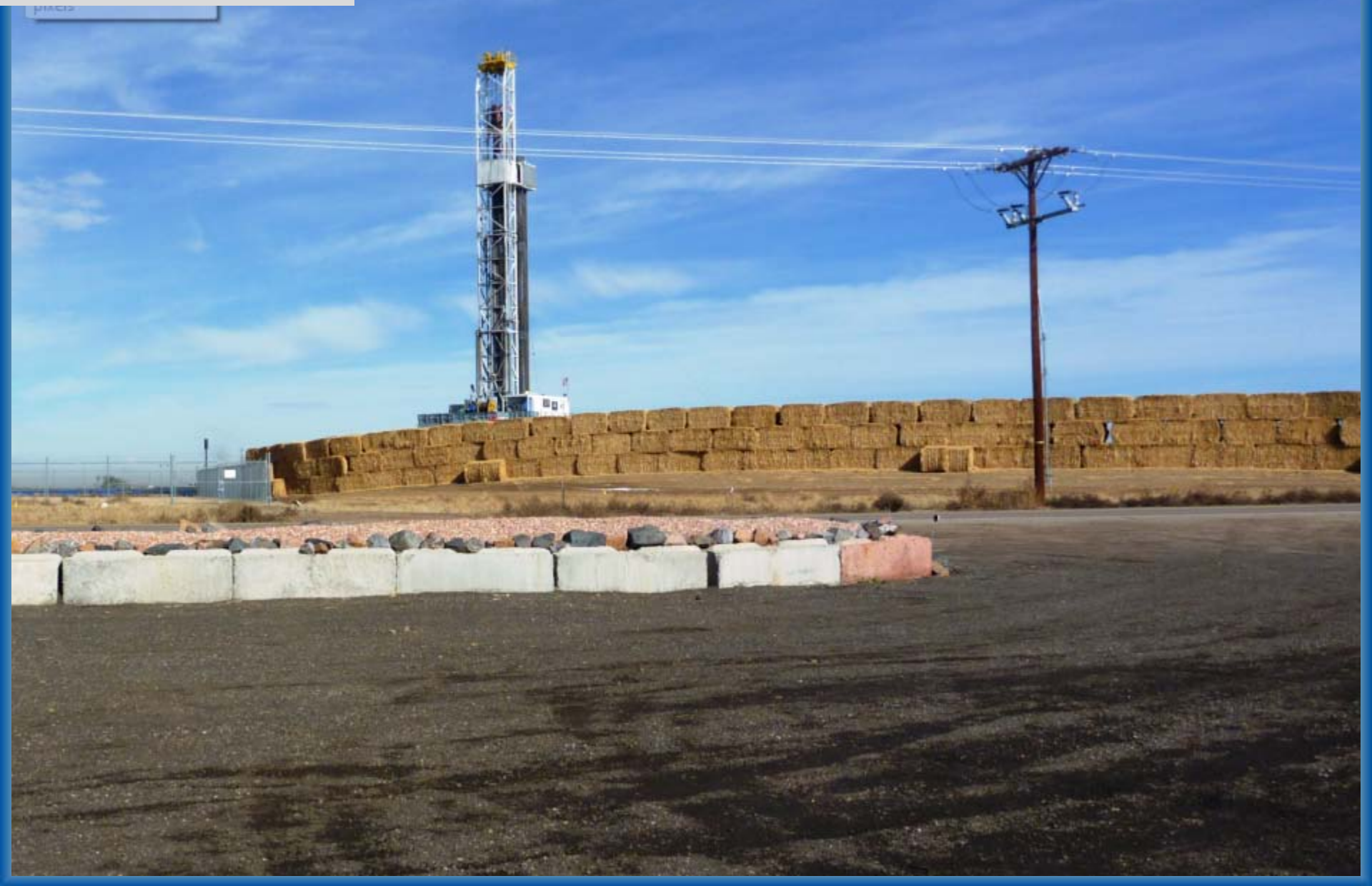
Temporary sound wall mitigating rig noise – Hay Bales
