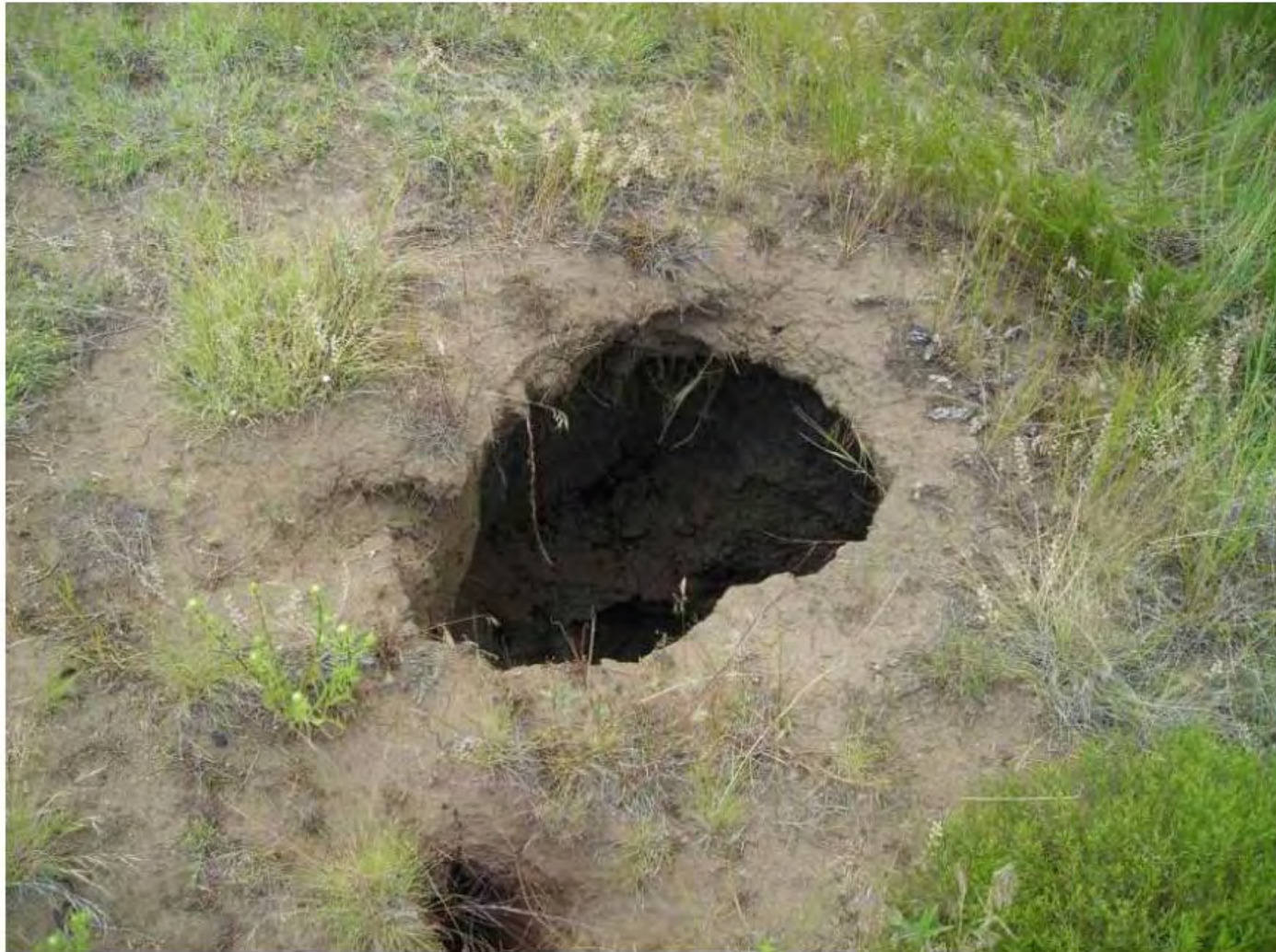
Sinkhole East of Apogee 640
