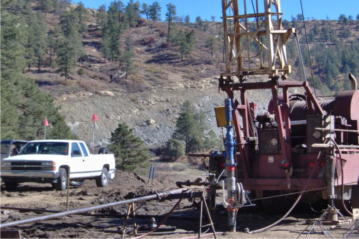
Photo 17: View of perforating operations at the Wagon Gulch site.
