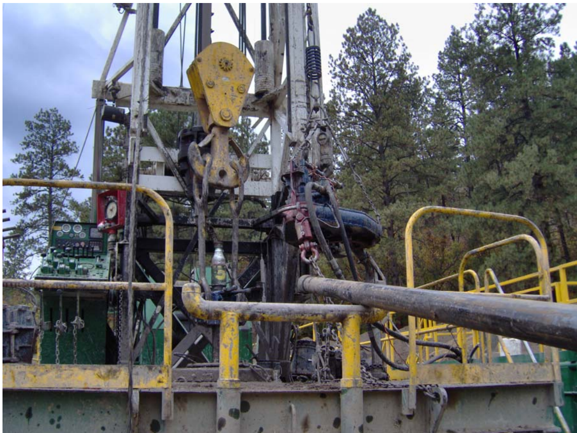
Photo 14: View of 4.5" steel casing installation at the Wagon Gulch site.
