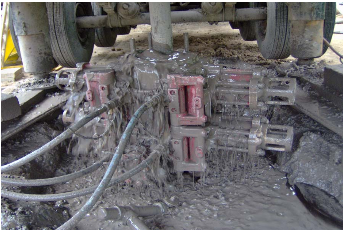
Photo 16: View of cementing operations at the Wagon Gulch site.
