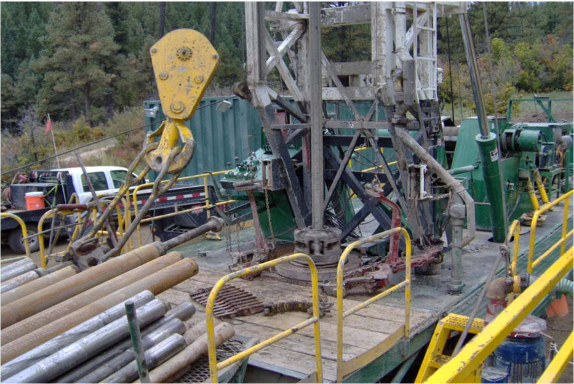
Photo 4: View of drilling operations at the Wagon Gulch site.
