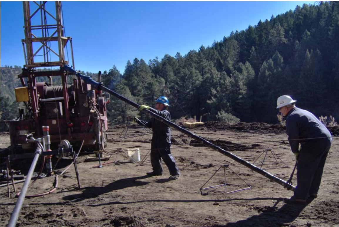
Photo 18: View of perforating operations at the Wagon Gulch site.
