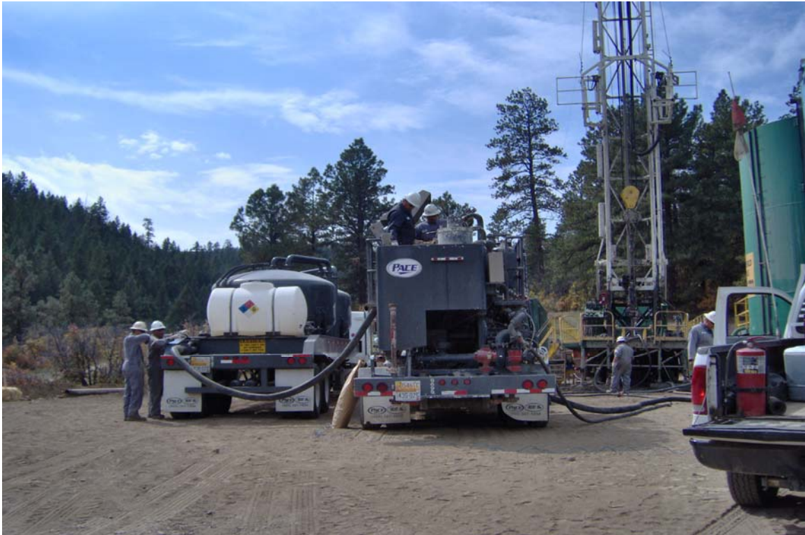
Photo 15: View of cementing operations at the Wagon Gulch site.
