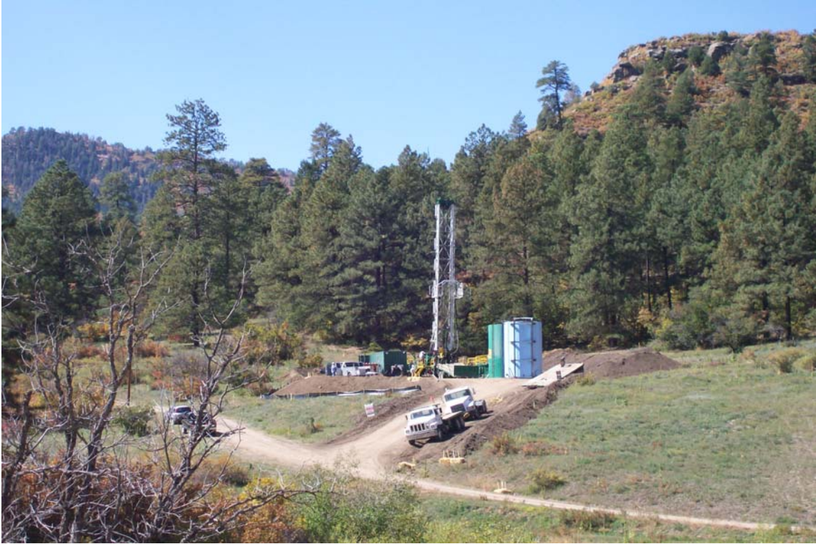
Photo 3: View of drilling operations at the Wagon Gulch site.
