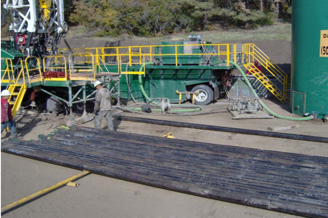
Photo 13: View of 4.5" steel casing at the Wagon Gulch site
