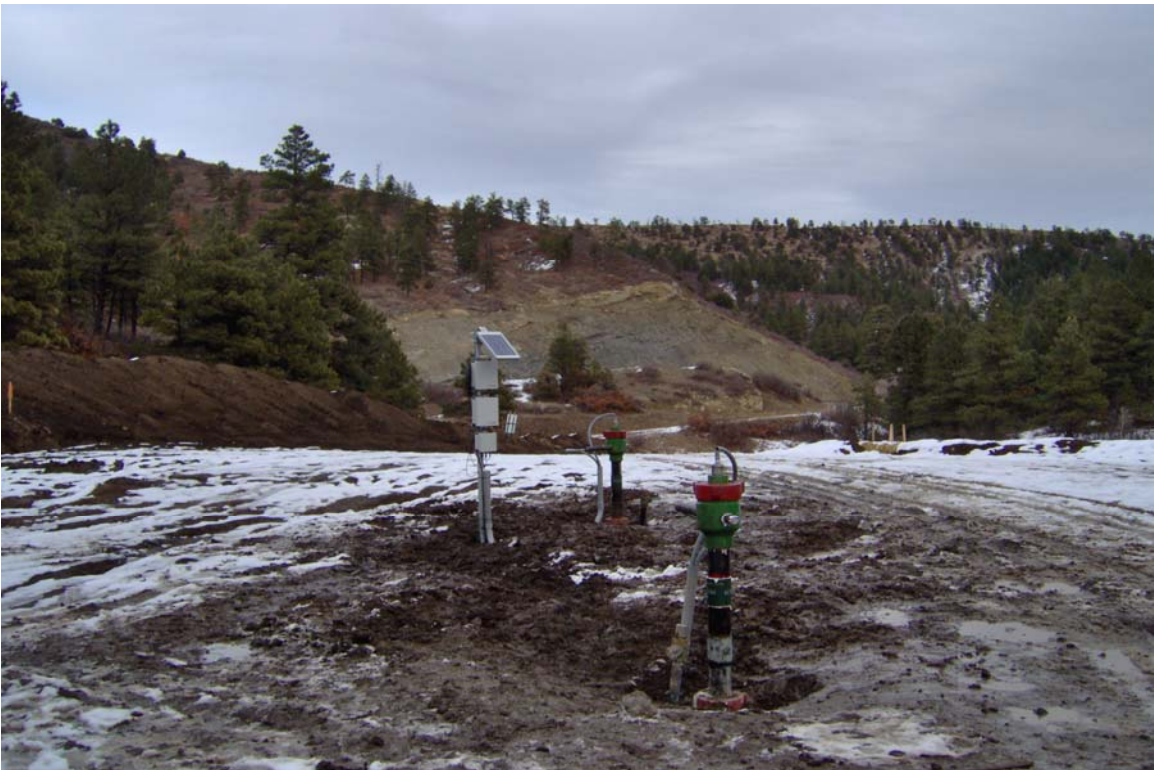
Photo 22: View of telemetry system installation the Wagon Gulch site
