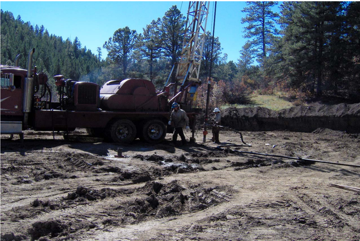
Photo 20: View of swabbing operations at the Wagon Gulch site.
