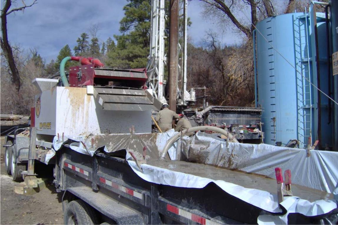
**Photo 15: View of conductor casing installation at the Palmer site.**
