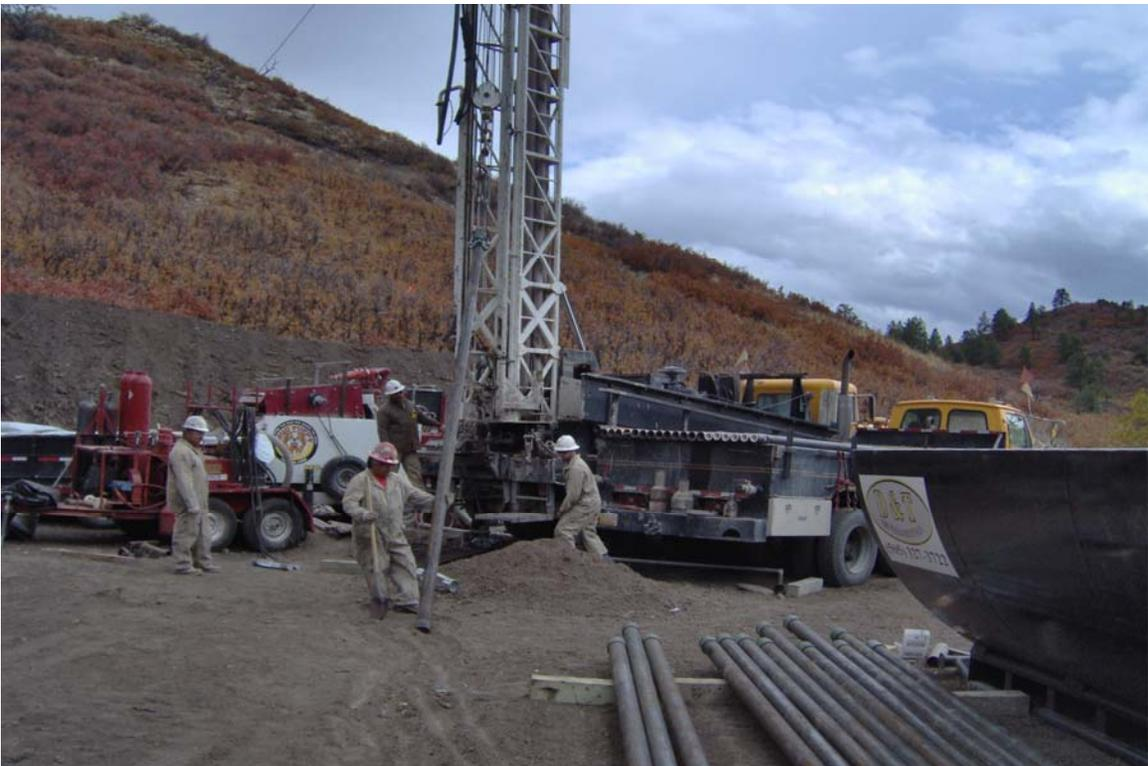
**Photo 6: View of 4.5" steel casing installation at the BP Highlands site.**
