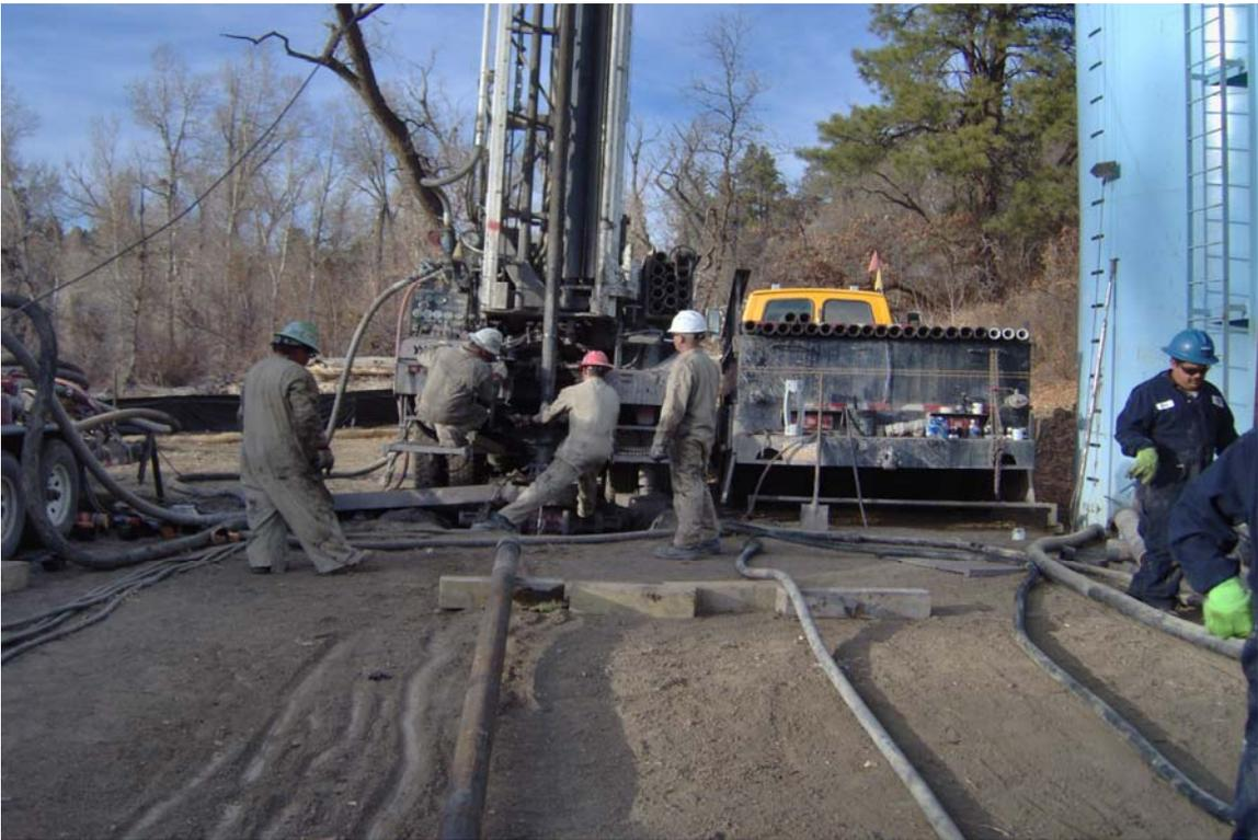
**Photo 20: View of installation of the 4.5" casing at the Palmer site.**
