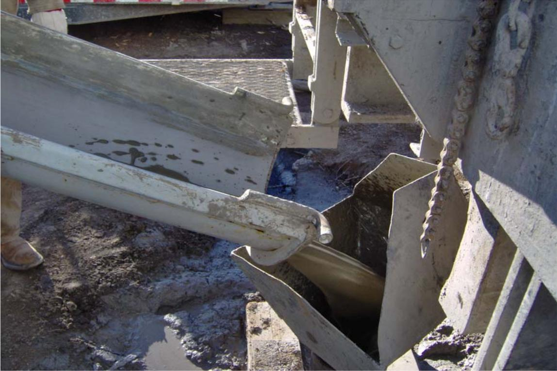
**Photo 19: View of cementing of the surface casing at the Palmer site.**
