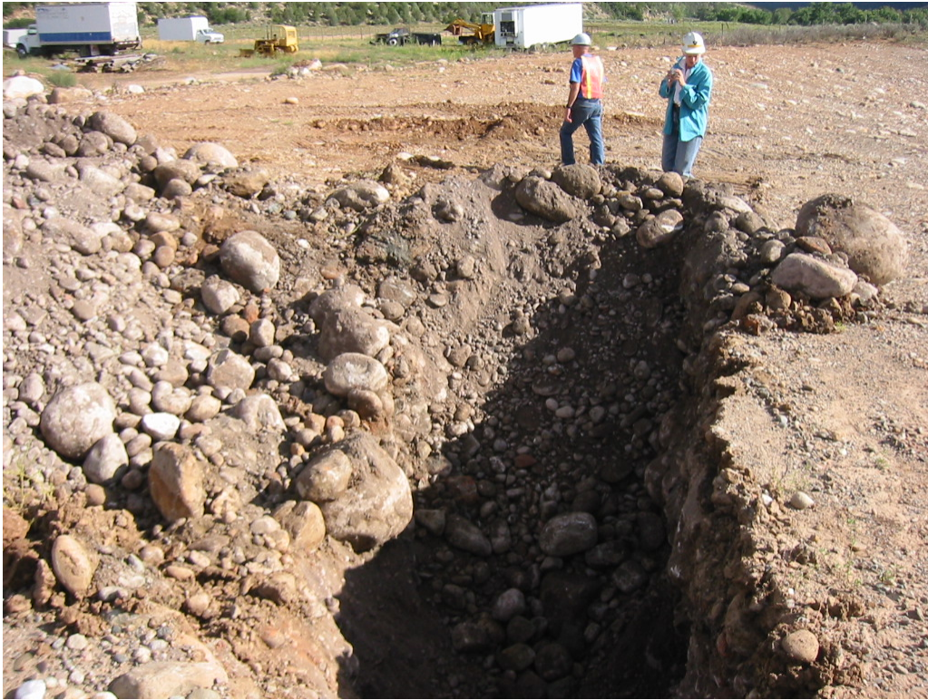
Photograph 5: Excavation at Anomaly #2, view south.
