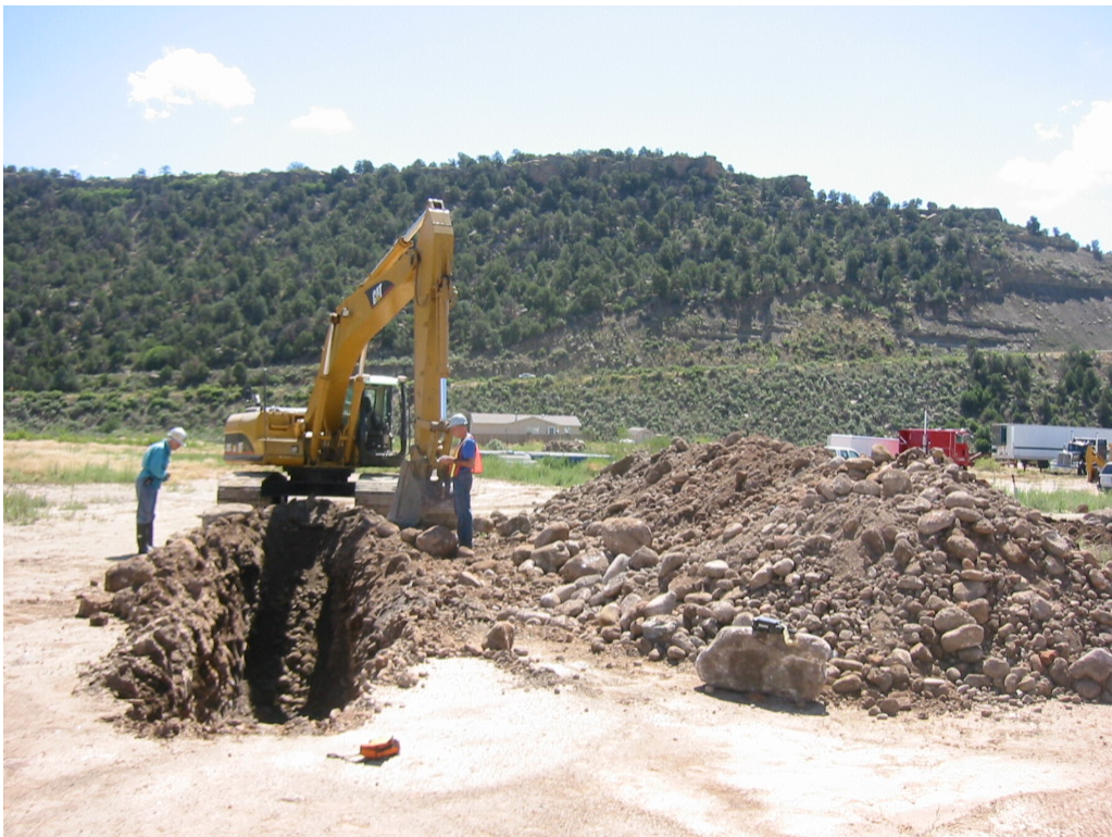
Photograph 4: Excavation at Anomaly #3, view east.
