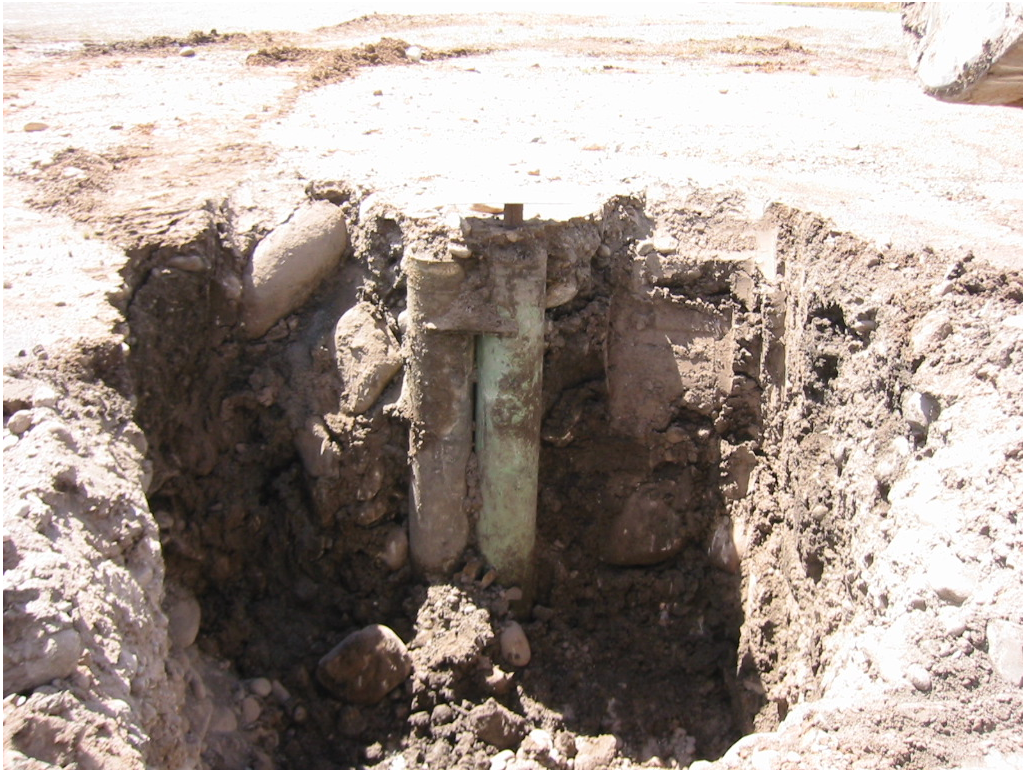
Photograph 1: NSBF #1 and “step-over” well, view north.
