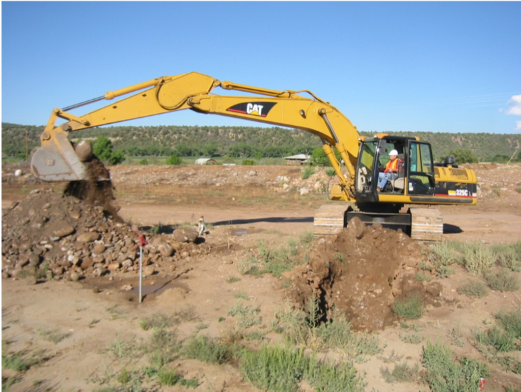
Photograph 3: Excavation at former Yoakum residence, view north.
