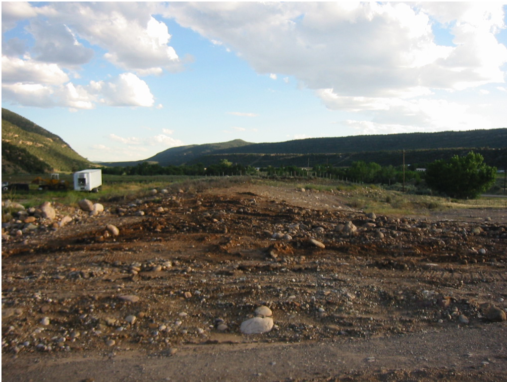
Photograph 6: Former Yoakum residence area following backfill, view south.
