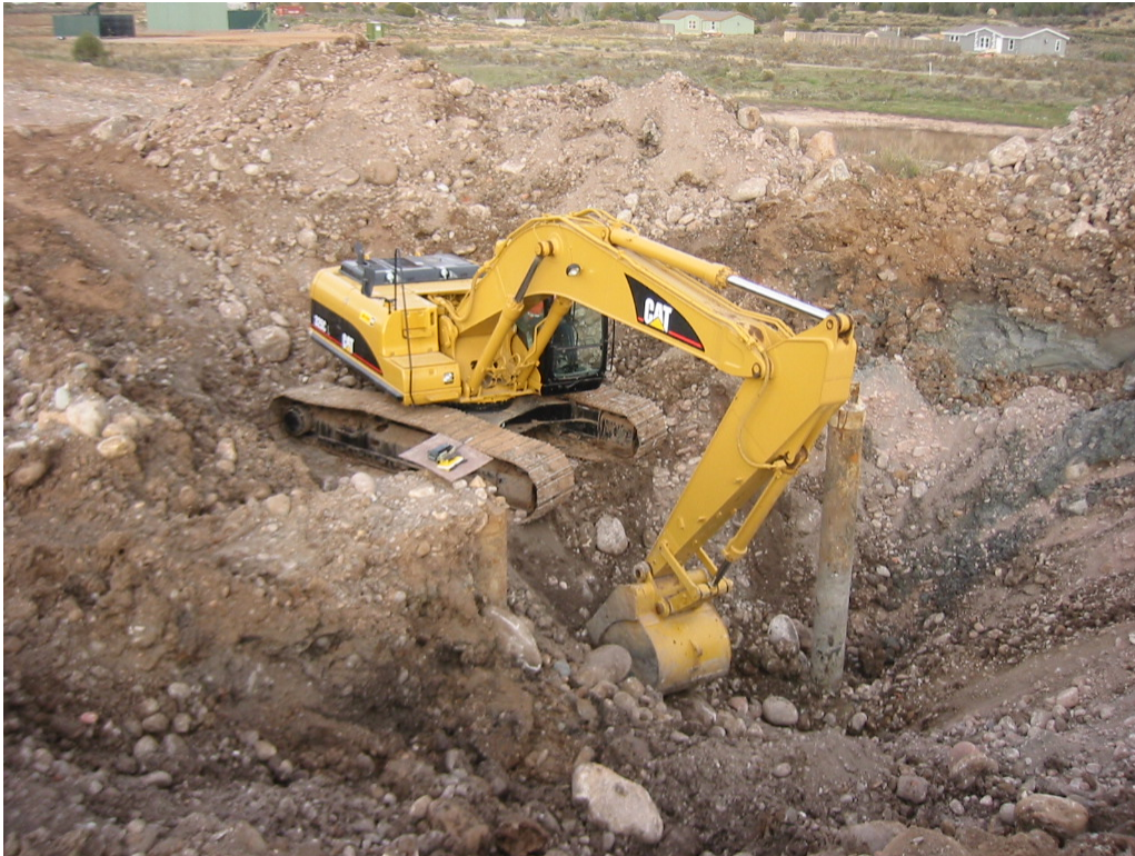
Photograph 1: Excavation of Bryce 1-X, view northeast.
