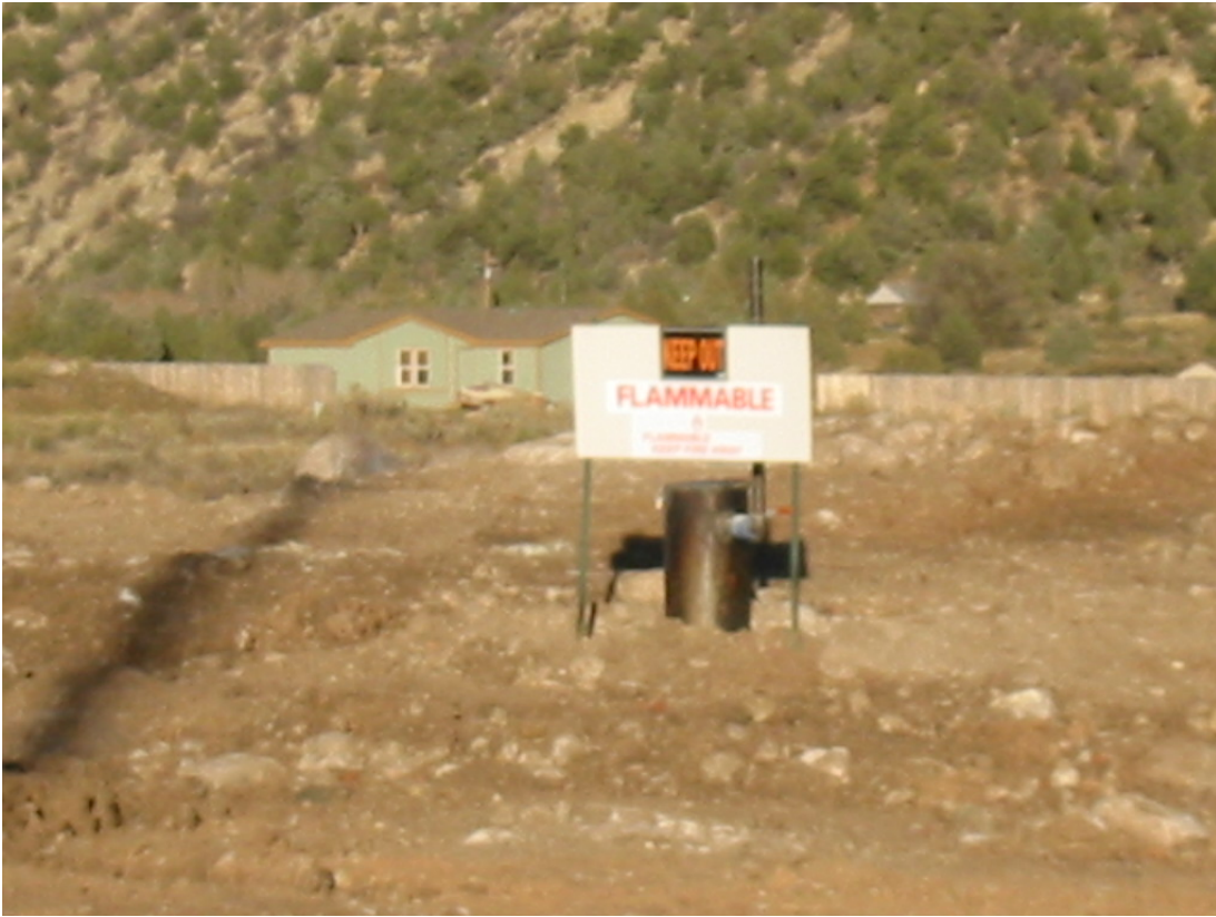
Photograph 14: Well head completion, view northeast.
