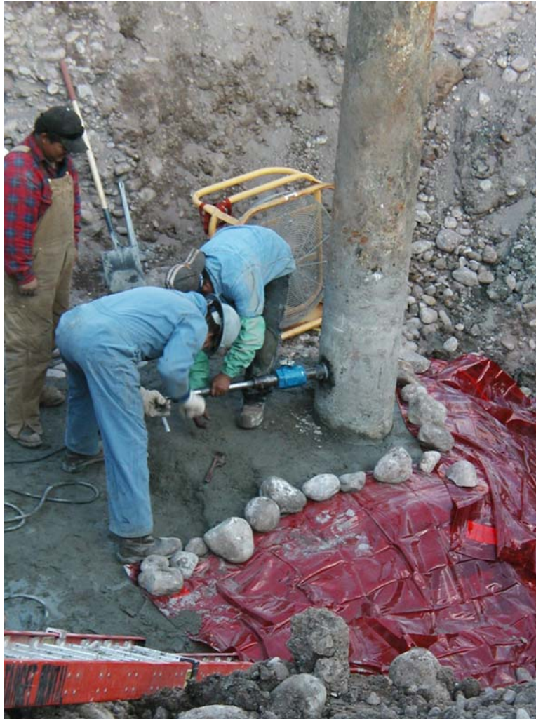
Photograph 7: Hot-tap with welding blanket barriers, view southeast.
