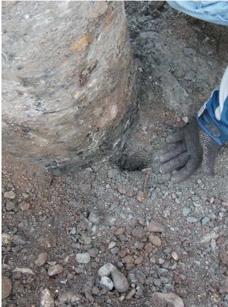
Photograph 3: Fracture in sandstone with seeping gas.
