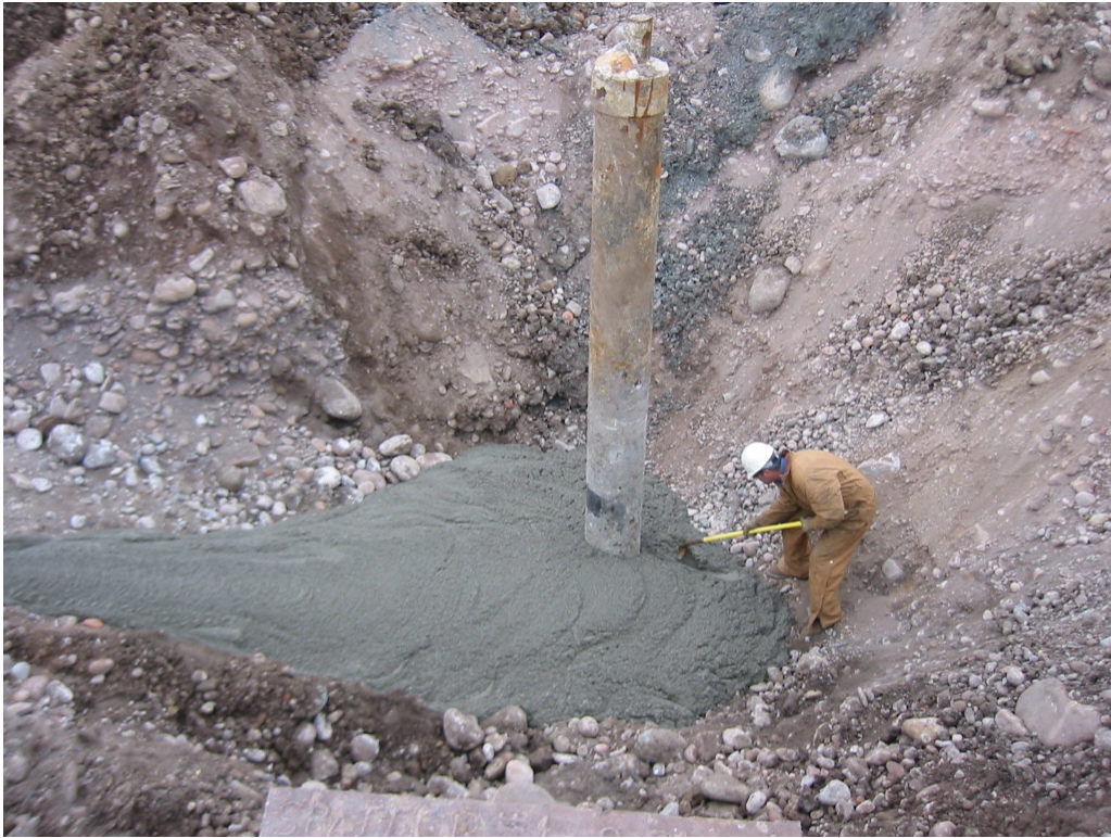
Photograph 5: Placement of concrete barrier, view east.
