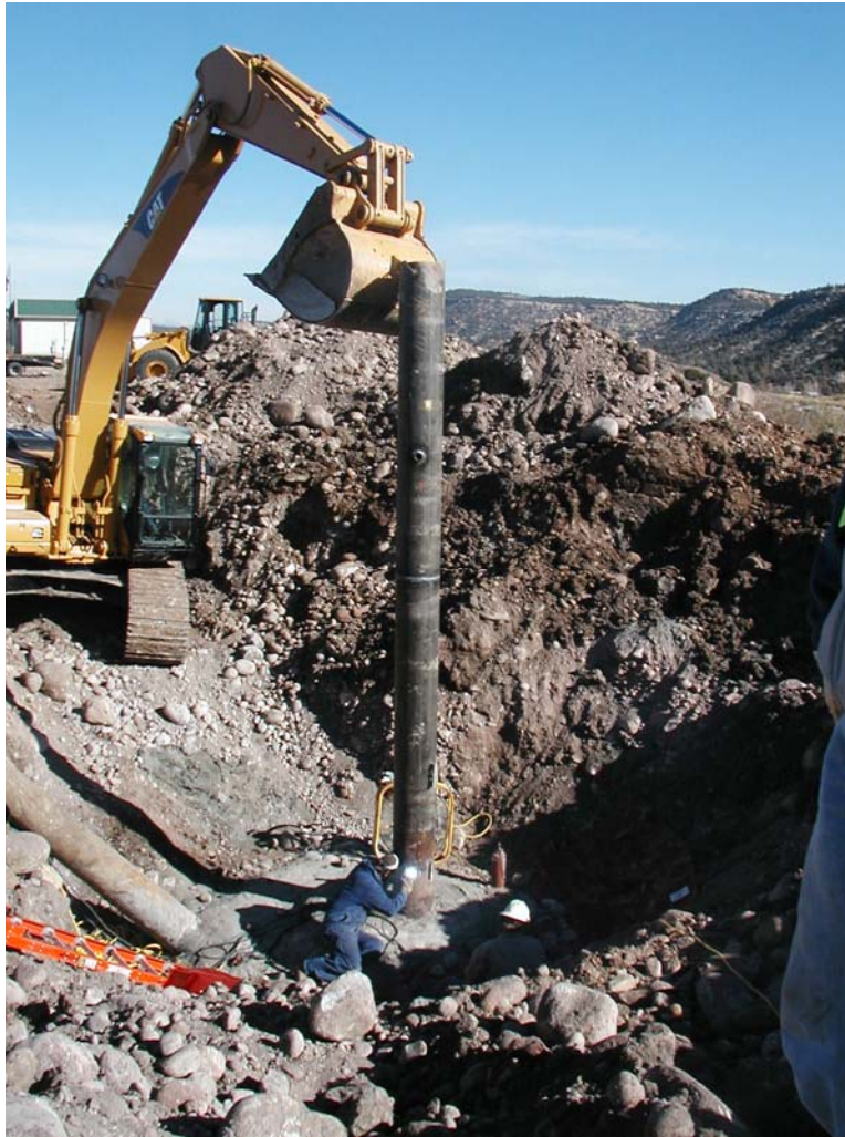
Photograph 10: Replacement of conductor pipe, view northeast.
