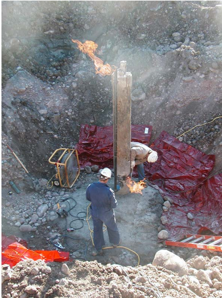
Photograph 8: Cut off of existing conductor pipe, view southeast.
