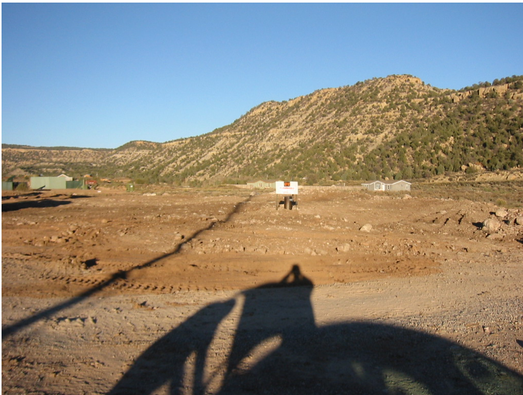
Photograph 13: Backfill of excavation area, view northeast.
