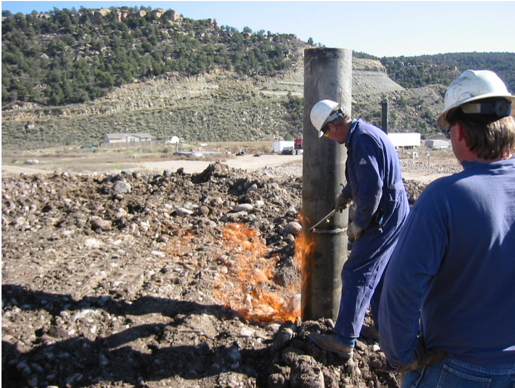
Photograph 12: Cutoff of conductor pipe at ground surface, view southeast.
