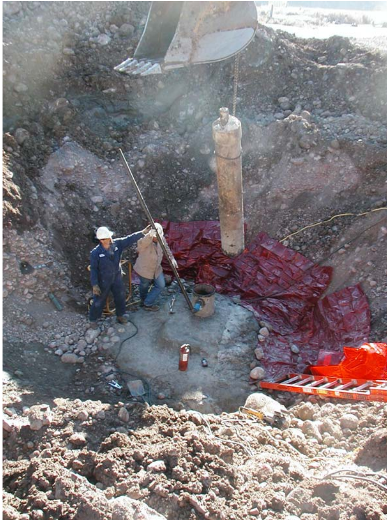
Photograph 9: Removal of existing conductor pipe, view southeast.
