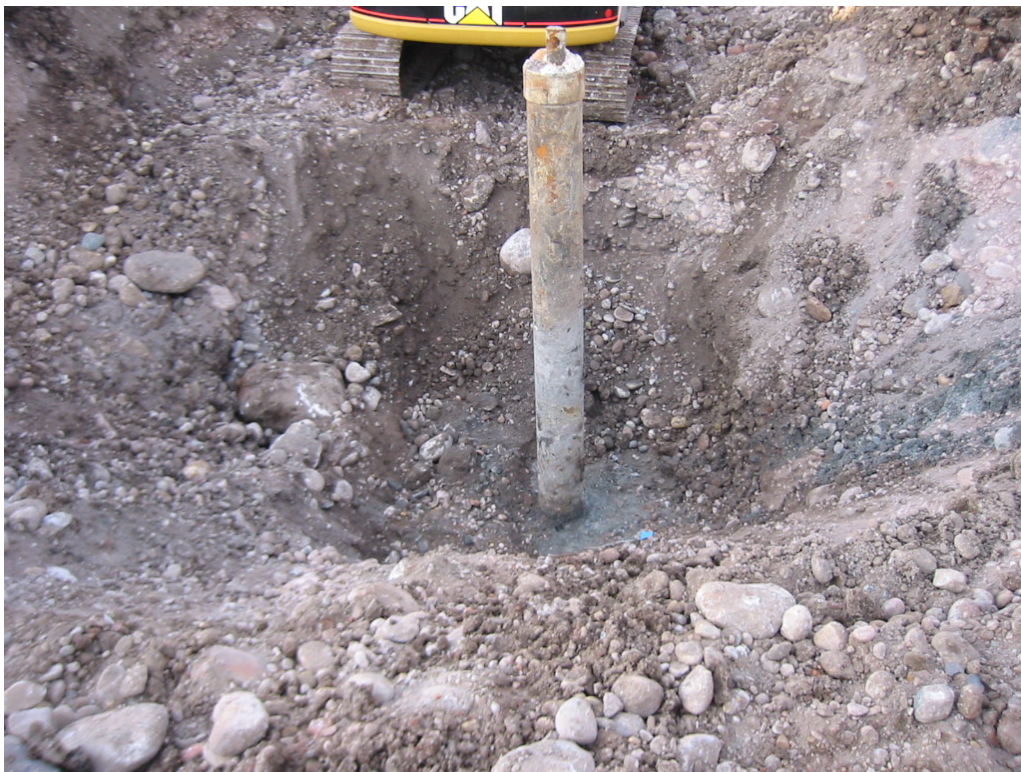
Photograph 2: Bryce 1-X excavation complete, note gray sandstone surface at bottom of conductor pipe, view north.
