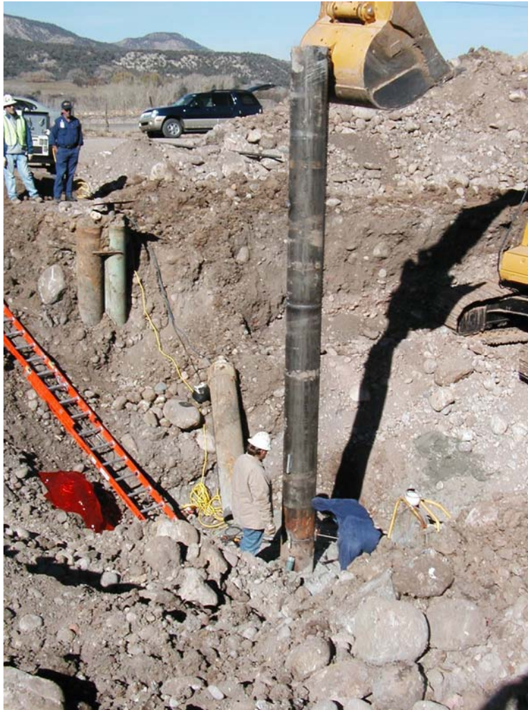
Photograph 11: Replacement of conductor pipe, view northwest.
