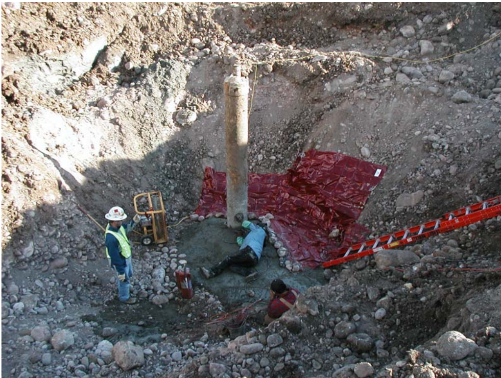
Photograph 6: Hot-tap with welding blanket barriers, view southeast.
