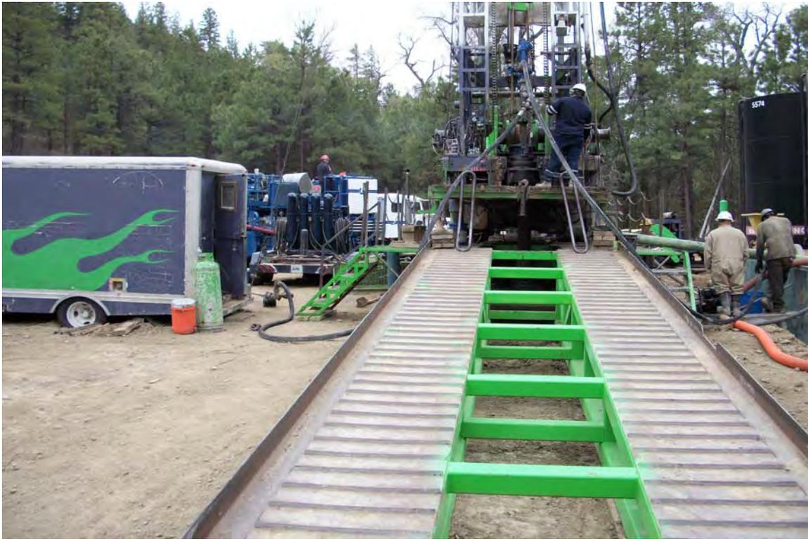
Photo 9: View of the cementing operations for the 4.5" long string casing.+
