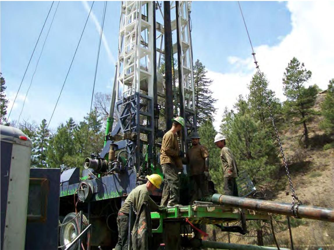
**Photo 6: View of 7" surface casing installation.**
