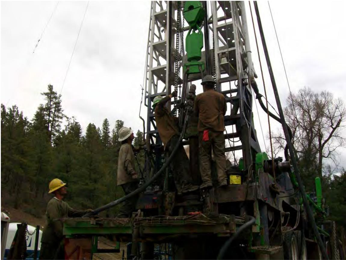
**Photo 7: View of the cementing operations for the 7" surface casing.**
