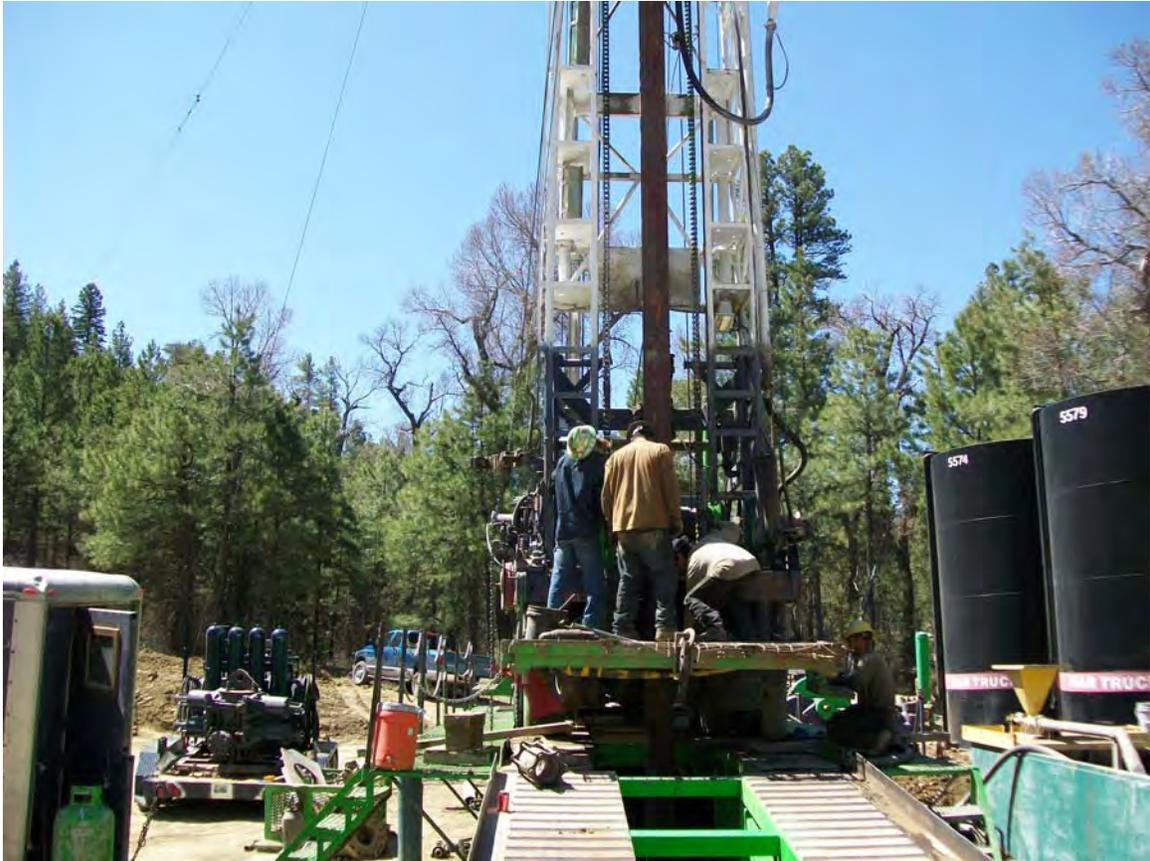
**Photo 3: View of 9 5/8" conductor casing installation.**
