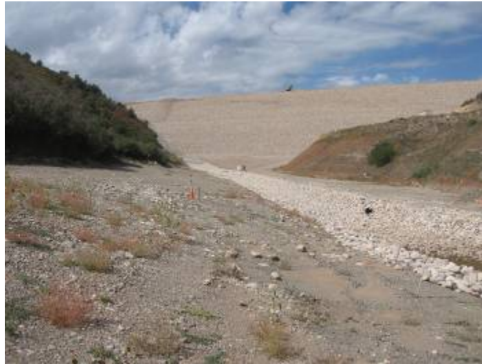
Construction activities at Basin Creek, view northeast.
