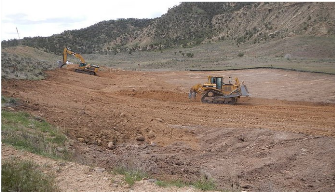
Figure 1: The COGCC's contractor recontours 4.5 acres of the location in 2015.
