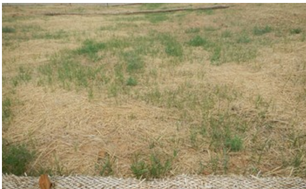
Access road area after restoration, revegetation germination and stabilization in August 2015
